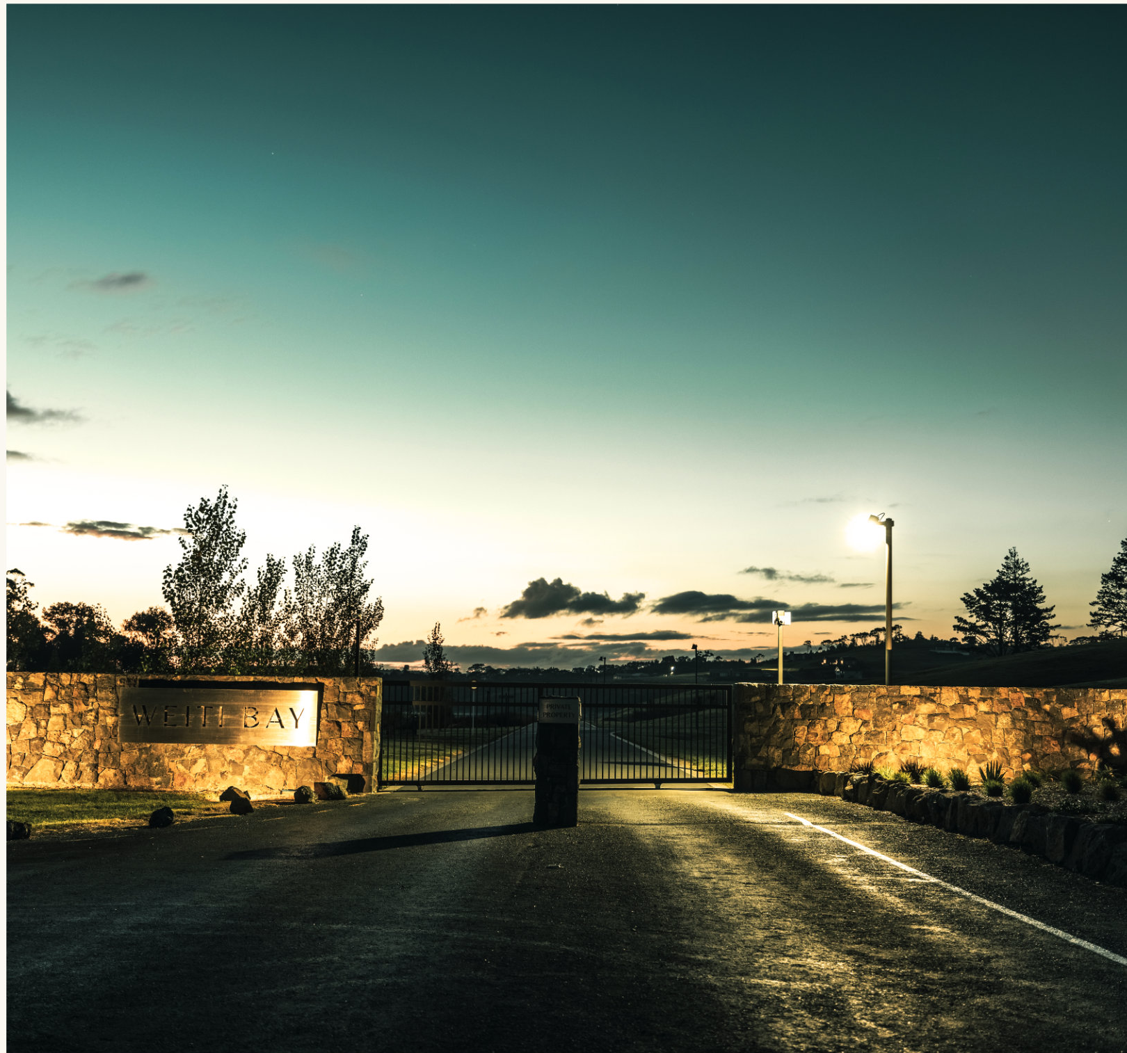
3.0 Weiti Bay | Entry to gated community
